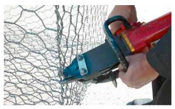
Figure 5B: The lacing process
